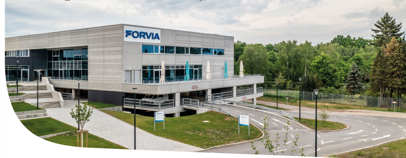
FORVIA Technology & Customer Center - Hanover, Germany
